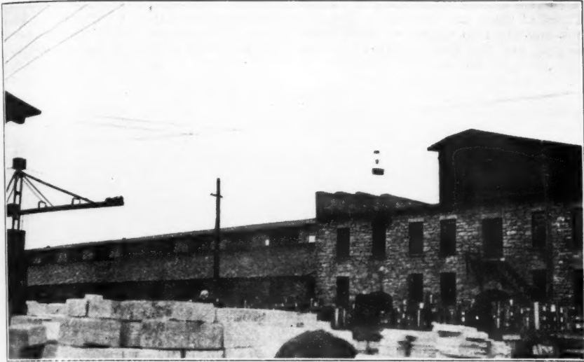
View Showing Shed on Top of Building Where Some of Sand Is Dumped
